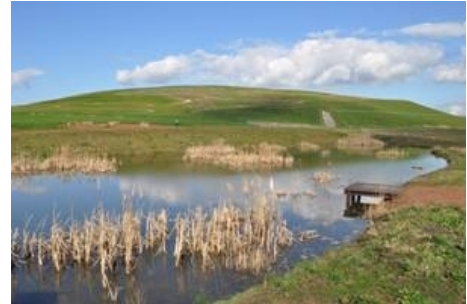
Picture 22 Example of a balancing pond
