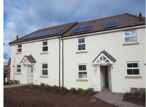
Picture 12 Photo-voltaic roof panels
