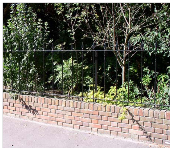
Modern railing, a boundary finish in keeping with the character of the village.
