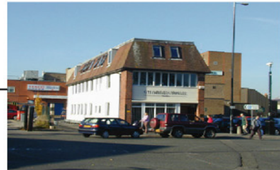
Charles Hoile Solicitor - small section of frontage onto Park Way
