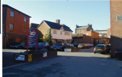
No. 2 and 3 (The Old St Nicholas Rectory) Grade II Listed early c.19th refronting of older building.
