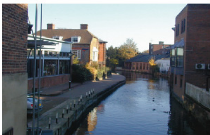
Mid-Georgian Old Rectory (waterside elevation) Two storeys. Double fronted with 3 windows. Hipped tile roof with 3 attic dormers.
