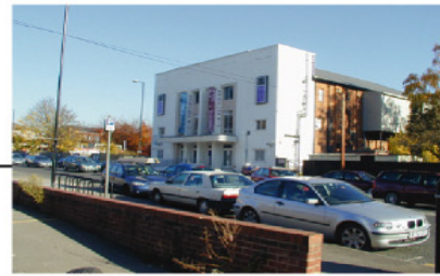
LA Fitness - former cinema at the entrance to Park Way
