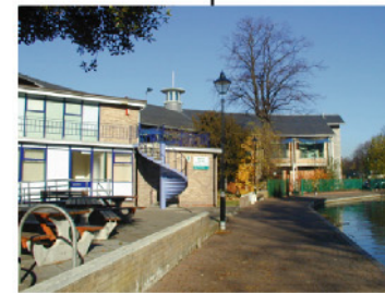
Opportunities to strengthen the canal walk and consider a pedestrian bridge crossing to permit a more circulatory flow around the Town Centre
