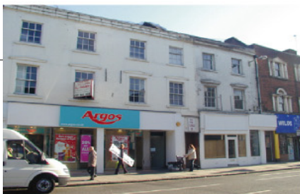
No. 36-37 (Argos) Grade II listed three storey early 19th century building. Slate and tile roofs. Stucco fronts with cornices. Recessed sash windows. Modern shop fronts.
