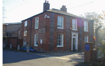
Marsh Cottage Grade II Listed early c.19th villa. Two storeys. Double-fronted with 3 windows. Hipped Welsh slate roof with brick stacks. Grey brick with red brick dressings.
