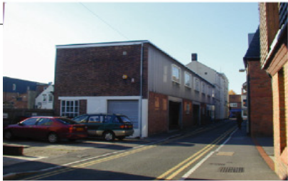
Poor quality office and warehouse units along Park Lane
