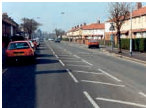
Fig. 10.2 Hatched road markings
