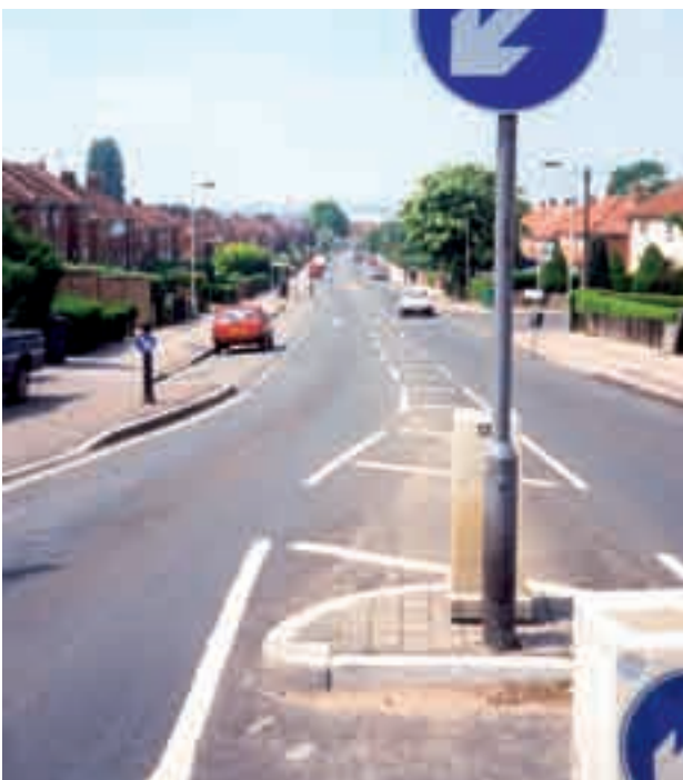
Fig. 2.5 Chicane of pedestrian refuge and sheltered parking
