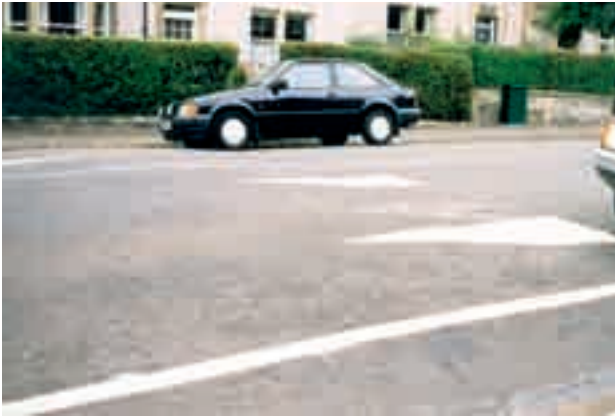
Fig 4.6 Sinusoidal road hump
