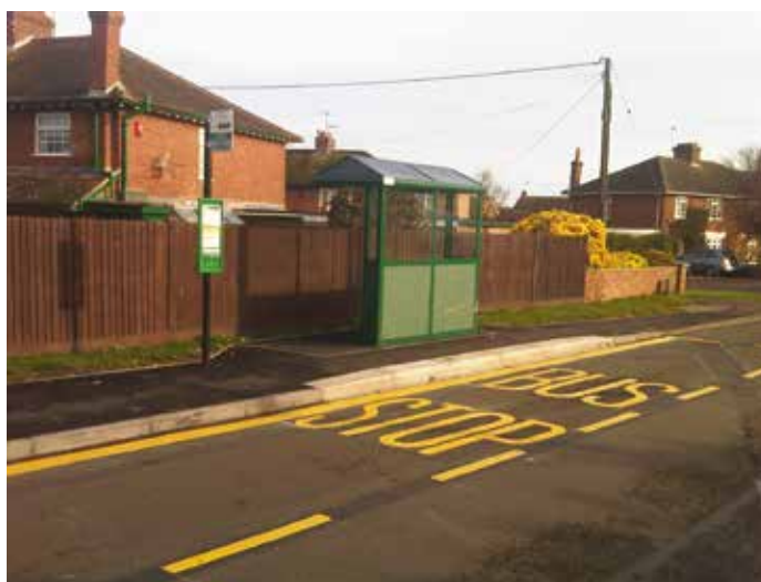
Figure 8.1: An example of an improved bus stop in Kintbury featuring new shelter, Kassel kerbing, pole and clearway.
