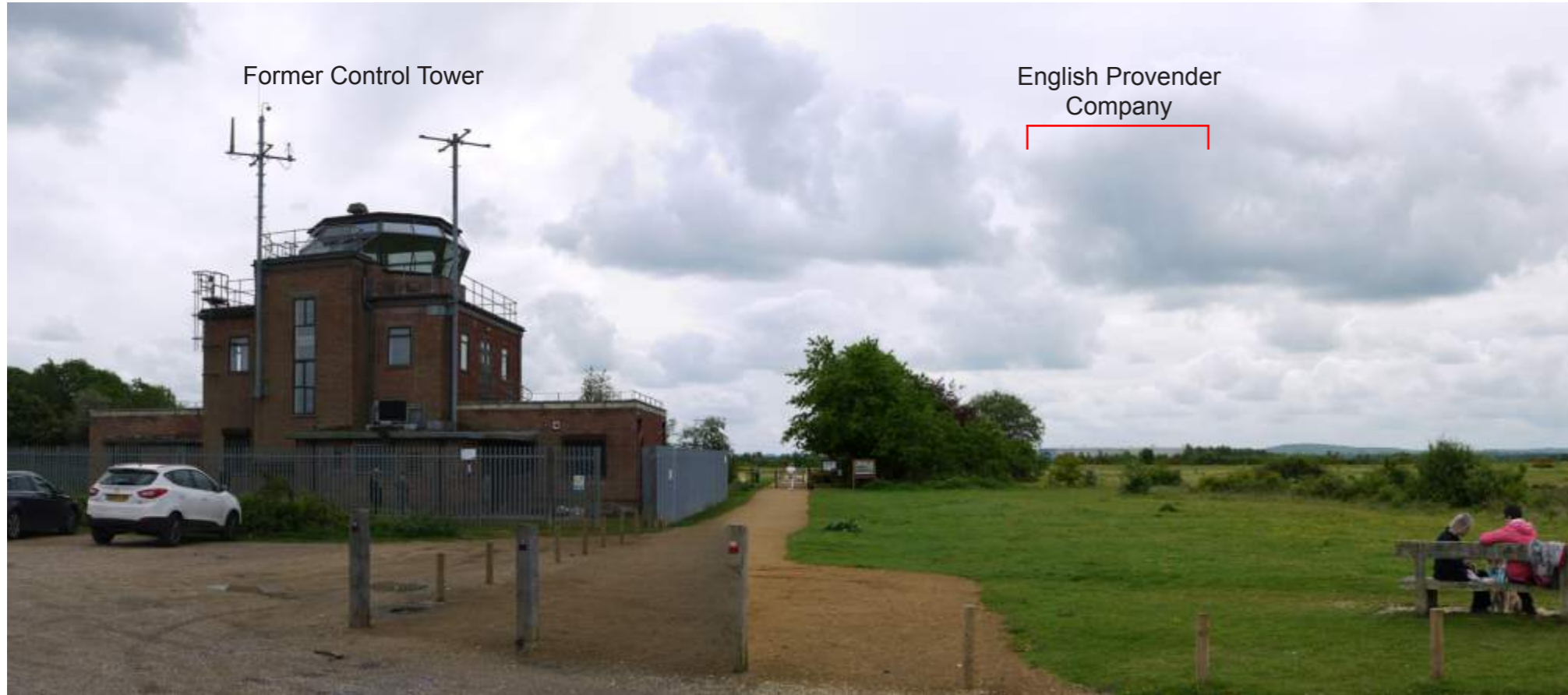
VP7 - View of Former Control Tower and south across the Common.
