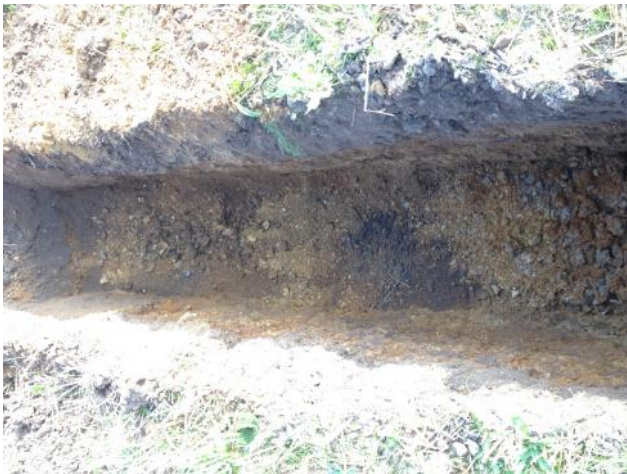
Photo 15: Excavation of trial pit TP07.
