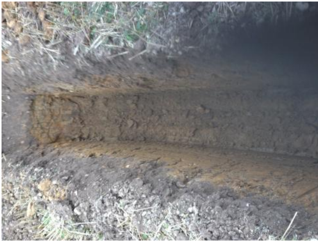
Photo 13: Excavation of trial pit TP06.
