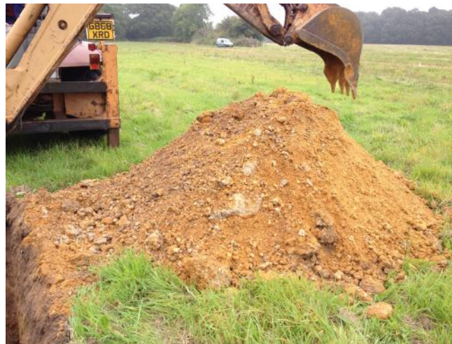
Photo 36: Arisings from trial pit TP16.
