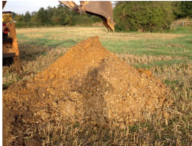
Photo 2: Arisings from trial pit TP01.
