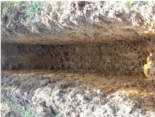
Photo 19: Excavation of trial pit TP08.
