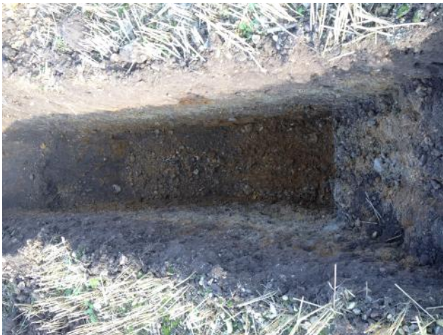
Photo 31: Excavation of trial pit TP14.
