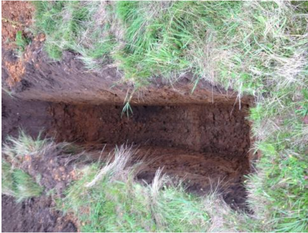
Photo 37: Excavation of trial pit TP17.
