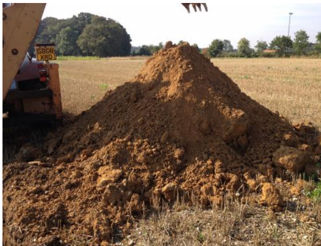
Photo 10: Arisings from trial pit TP05.
