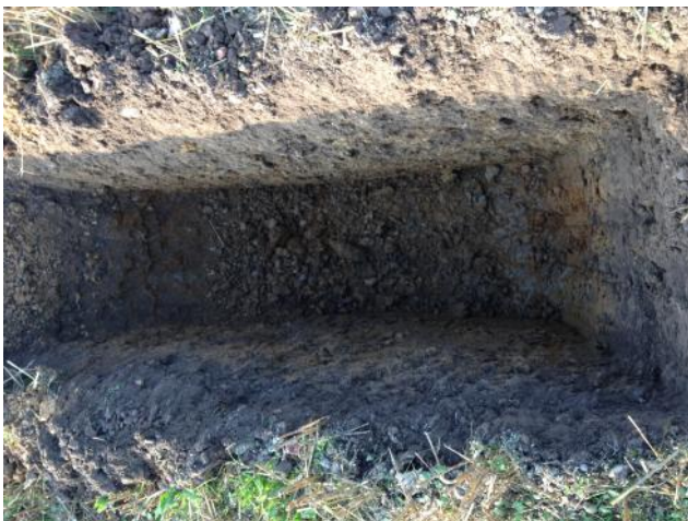
Photo 11: Excavation of trial pit TP05A.
