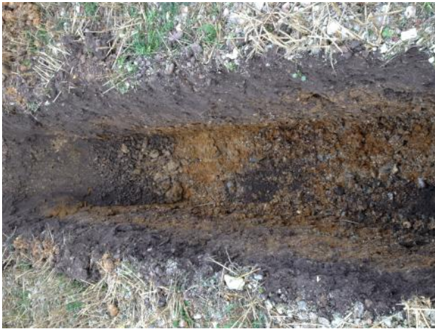
Photo 5: Excavation of trial pit TP03.
