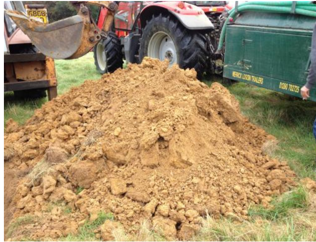
Photo 22: Arisings from trial pit TP09.
