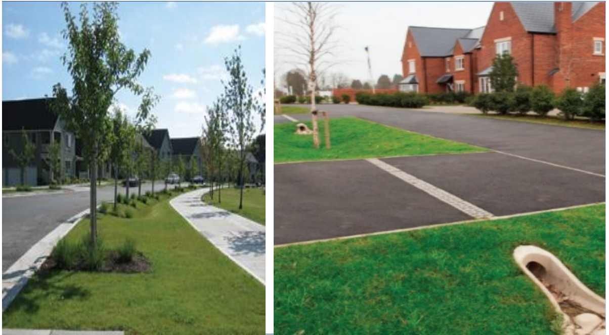
Figure 6-3: Swale along road corridor
