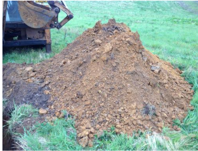
Photo 30: Arisings from trial pit TP13.
