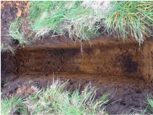
Photo 29: Excavation of trial pit TP13.
