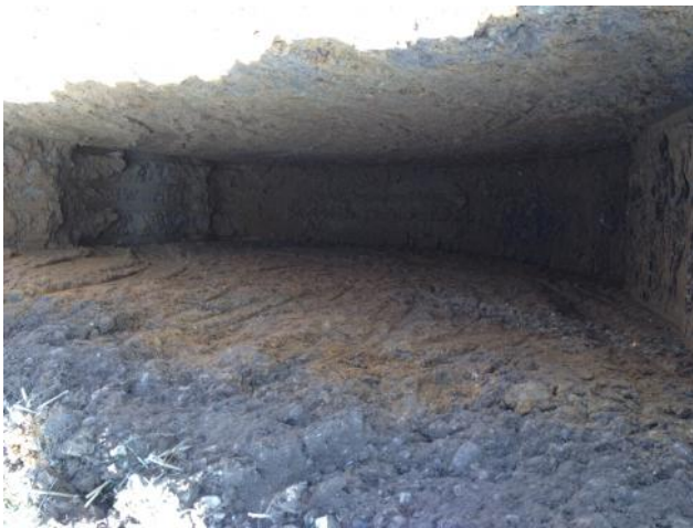
Photo 33: Excavation of trial pit TP15.
