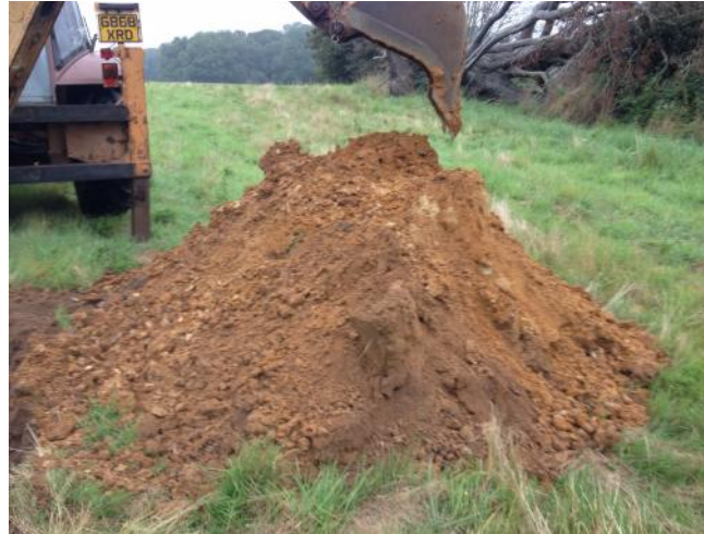
Photo 26: Arisings from trial pit TP11.
