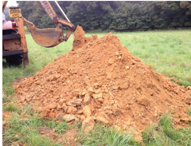
Photo 28: Arisings from trial pit TP12.
