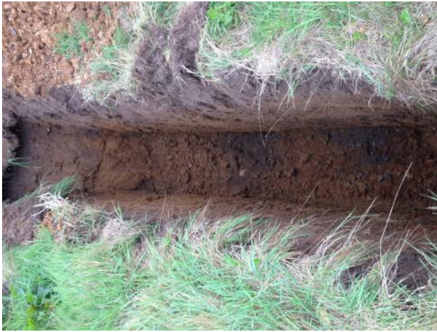
Photo 25: Excavation of trial pit TP11.
