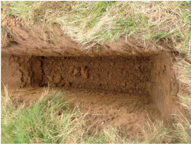
Photo 21: Excavation of trial pit TP09.
