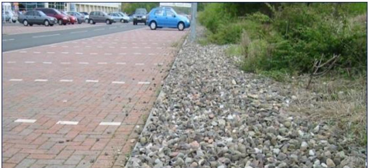
Figure 6-4: Filter Strip along highway
