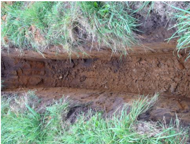
Photo 27: Excavation of trial pit TP12.
