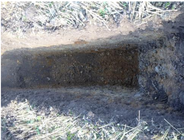
Photo 1: Excavation of trial pit TP01.
