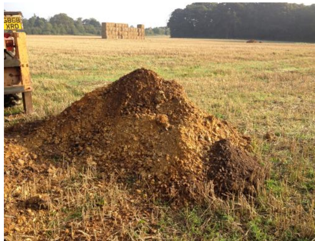
Photo 16: Arisings from trial pit TP07.
