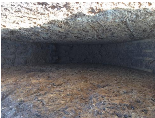
Photo 9: Excavation of trial pit TP05.
