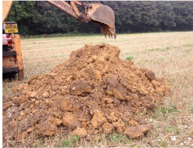
Photo 14: Arisings from trial pit TP06.
