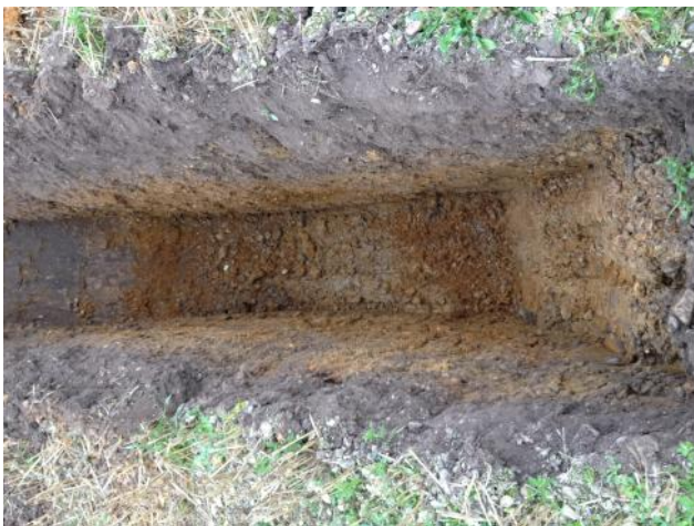
Photo 7: Excavation of trial pit TP04.
