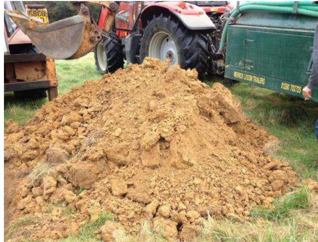
Photo 22: Arisings from trial pit TP09.
