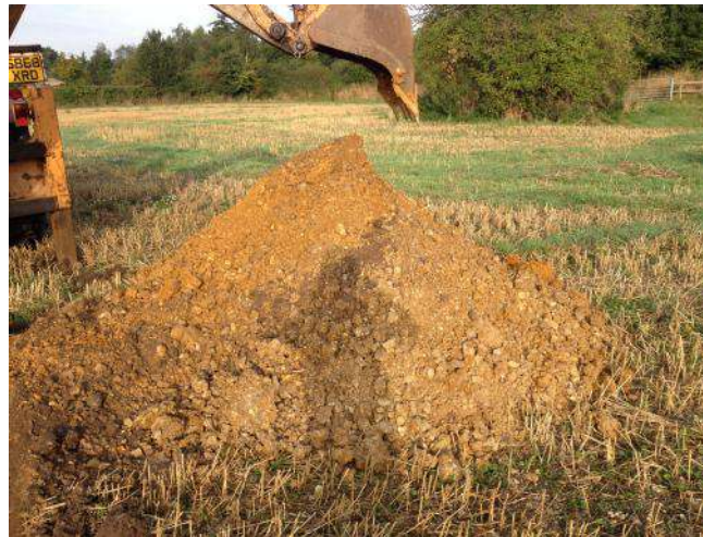
Photo 32: Arisings from trial pit TP14.
