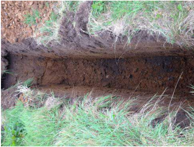
Photo 25: Excavation of trial pit TP11.
