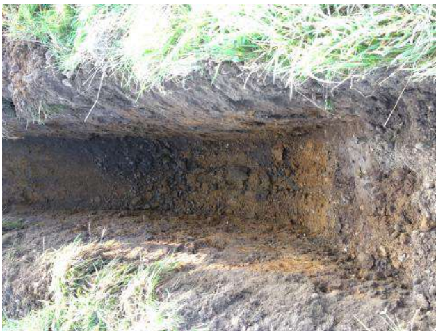
Photo 23: Excavation of trial pit TP10.
