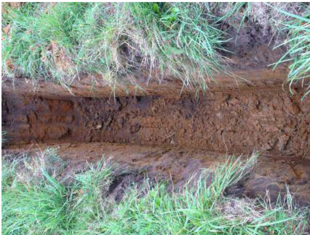
Photo 27: Excavation of trial pit TP12.
