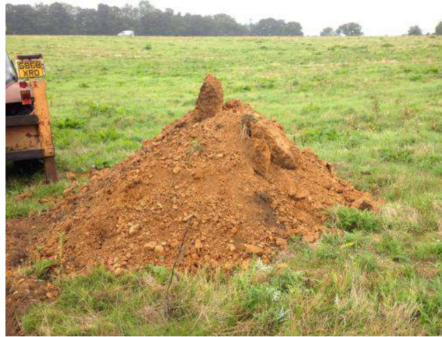
Photo 38: Arisings from trial pit TP17.
