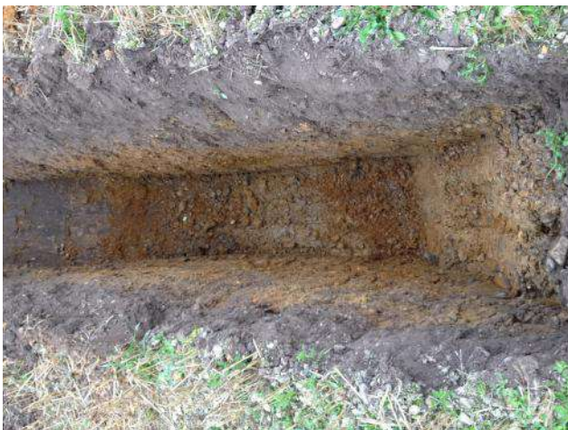
Photo 7: Excavation of trial pit TP04.
