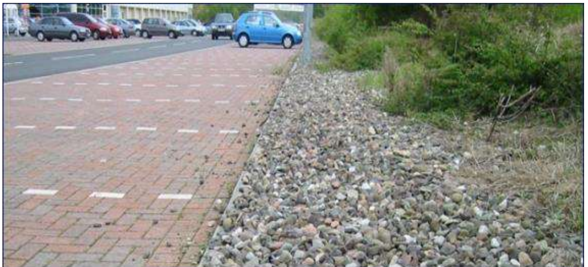
Figure 6-4: Filter Strip along highway
