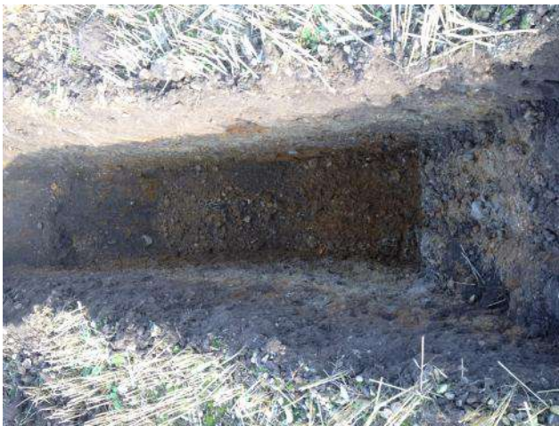
Photo 1: Excavation of trial pit TP01.
