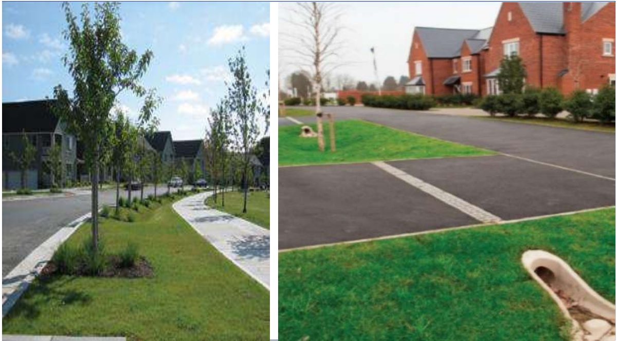
Figure 6-3: Swale along road corridor
