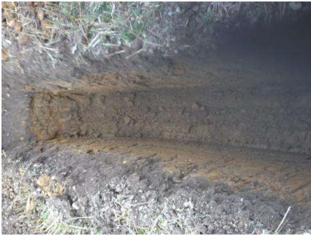
Photo 13: Excavation of trial pit TP06.
