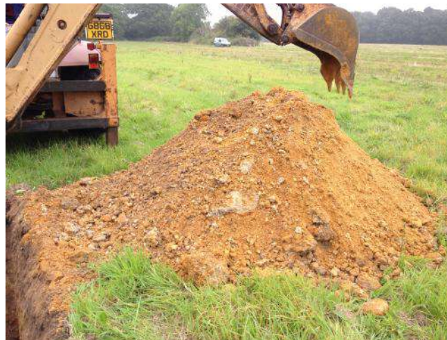
Photo 36: Arisings from trial pit TP16.
