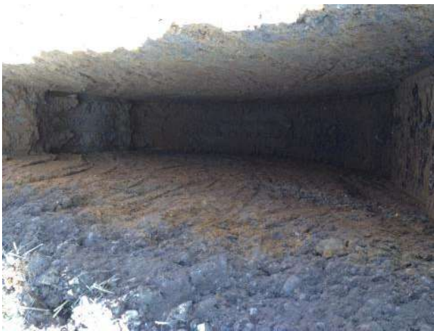
Photo 3: Excavation of trial pit TP02.
