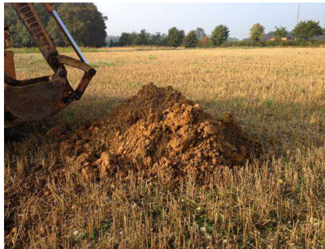
Photo 12: Arisings from trial pit TP05A.
