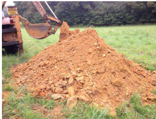
Photo 28: Arisings from trial pit TP12.
