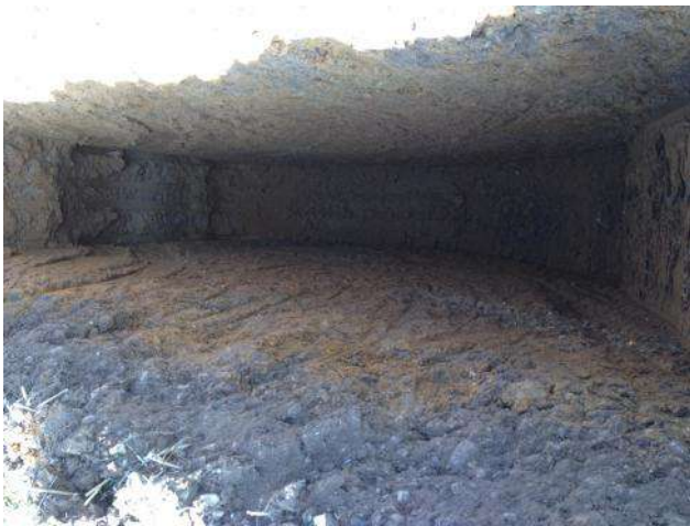
Photo 33: Excavation of trial pit TP15.
