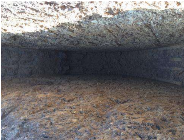
Photo 9: Excavation of trial pit TP05.
