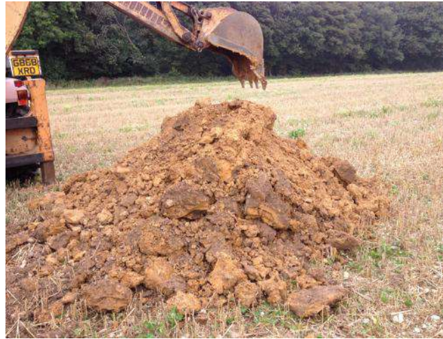
Photo 14: Arisings from trial pit TP06.
