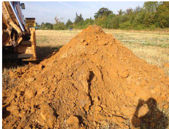
Photo 4: Arisings from trial pit TP02.
