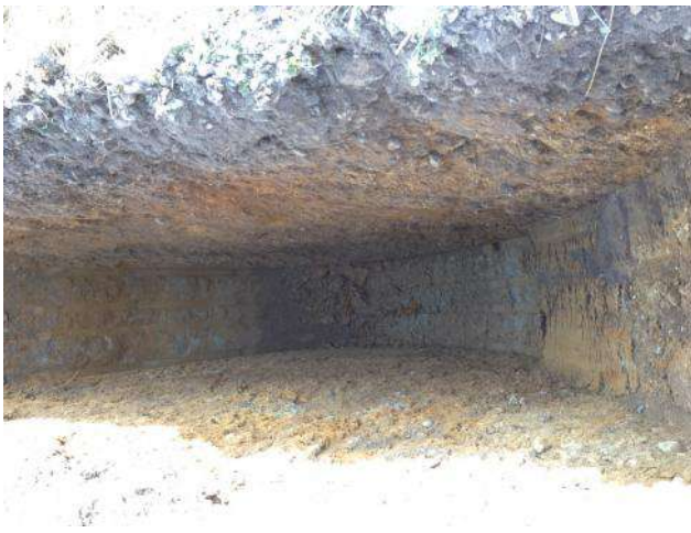
Photo 17: Excavation of trial pit TP07A.
