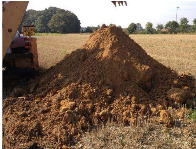
Photo 10: Arisings from trial pit TP05.
