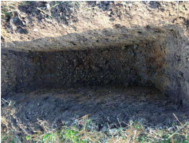
Photo 11: Excavation of trial pit TP05A.
