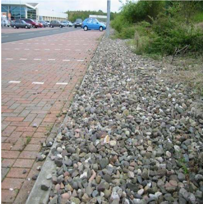
Figure 4e: Filter Strip along highway
