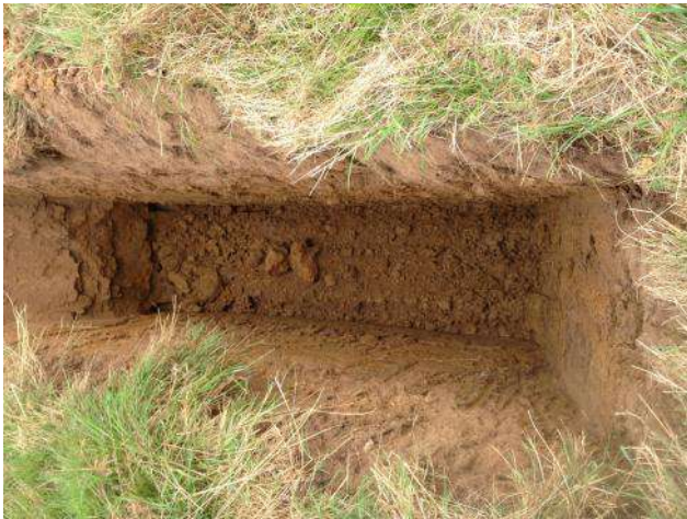
Photo 21: Excavation of trial pit TP09.
