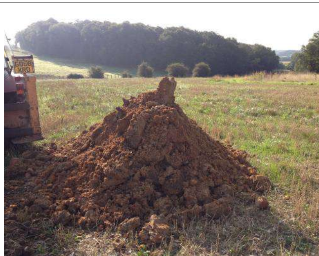
Photo 20: Arisings from trial pit TP08.
