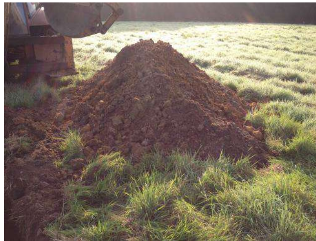
Photo 24: Arisings from trial pit TP10.
