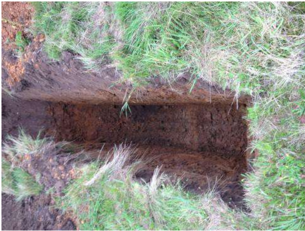
Photo 37: Excavation of trial pit TP17.
