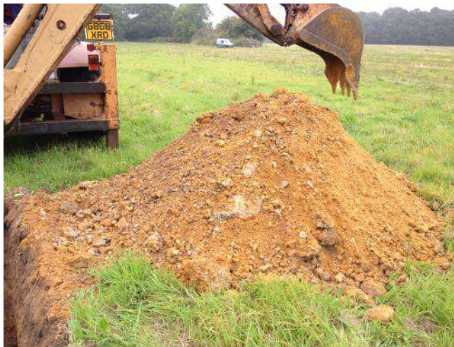
Photo 36: Arisings from trial pit TP16.
