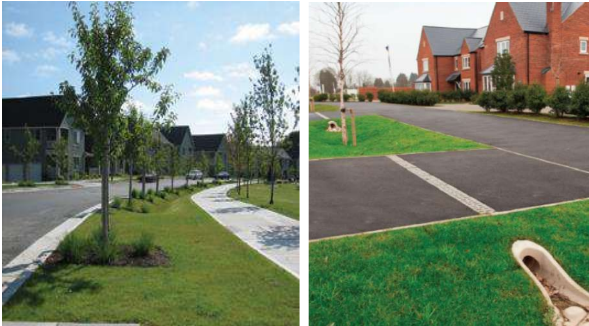
Figure 4d: Swale along road corridor
