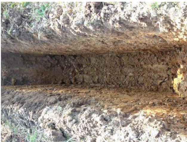
Photo 19: Excavation of trial pit TP08.
