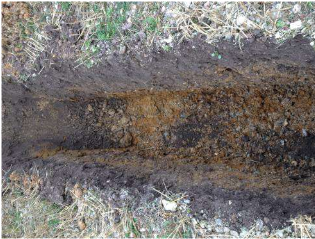
Photo 5: Excavation of trial pit TP03.
