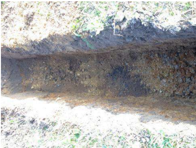
Photo 15: Excavation of trial pit TP07.
