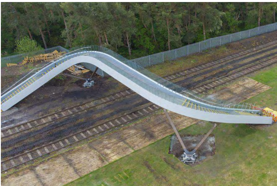
Image 3.2: Flow Bridge Railway Crossing
