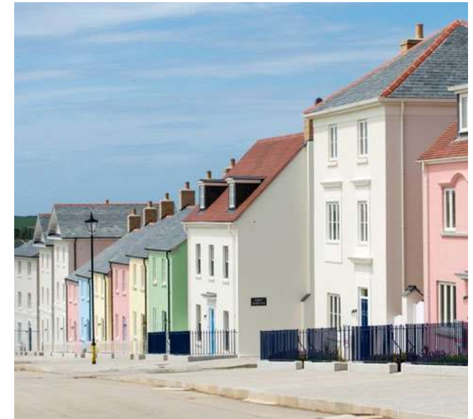
A wide street with house frontages stepping down along its length. Their simple forms, considered roof detailing, and colourful façades create a strong identity appropriate to the local and wider context of Nansledan, Newquay.
