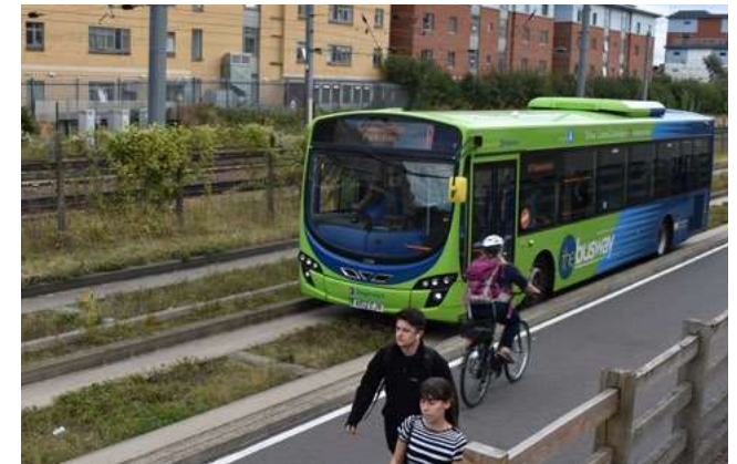
A guided busway with dedicated pedestrian and cycle paths provides fast and direct links to connect new and existing neighbourhoods with employment and services in Cambridgeshire.
