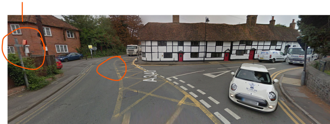
Figure 3- Clear signposts to danger of the Pangbourne Hill junction- tyre marks for wide swinging vehicles using 'wrong' carriageway and also mirror
